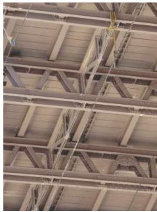
Late 19th century bridge construction made up of a myriad of smaller pieces of steel, which made coating application extra challenging.
