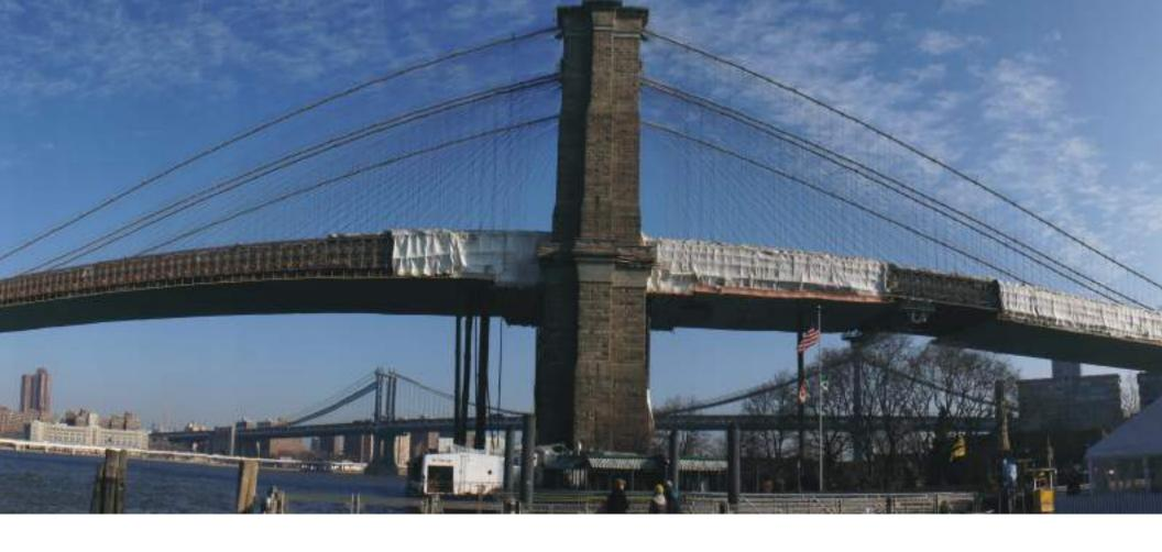
As the oldest suspension bridge in active use in America, the Brooklyn Bridge recoating project required a complex strategy to match the complex conditions of the task at hand.
