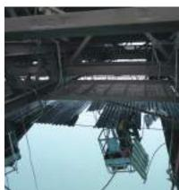
A non-project associated barge and the crane it was transporting struck the underbridge platform, fortunately causing no injuries, but created a 50-foot-wide (15m) gash which snapped numerous platform support cables, again causing an adverse effect on the CPM; removal of the platform for repair was done as an emergency condition under coordination with the Office of Emergency Management and in conjuction with the SafeSpan design engineer.
