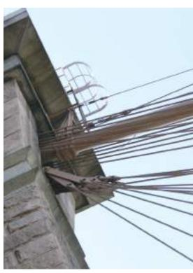
Approximately 4.2 million square feet (390,193m2) of steel beams, braces and cables of the bridge, as well as the Manhattan and Brooklyn ramps – essentially the structural "bones" – were specified for a coatings overhaul.
