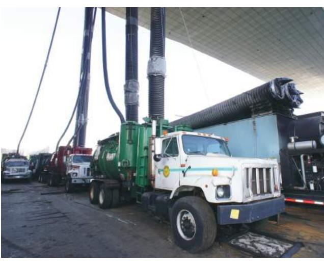
Lead-based paint removal required complete "cradle to grave" handling of hazardous wastes, with equipment situated over 1,200 feet away from the class 1A containment due to weight limitations of the structure and roadway closure limitations.
