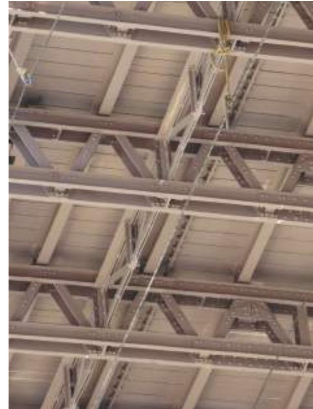
Late 19th century bridge construction made up of a myriad of smaller pieces of steel, which made coating application extra challenging.
