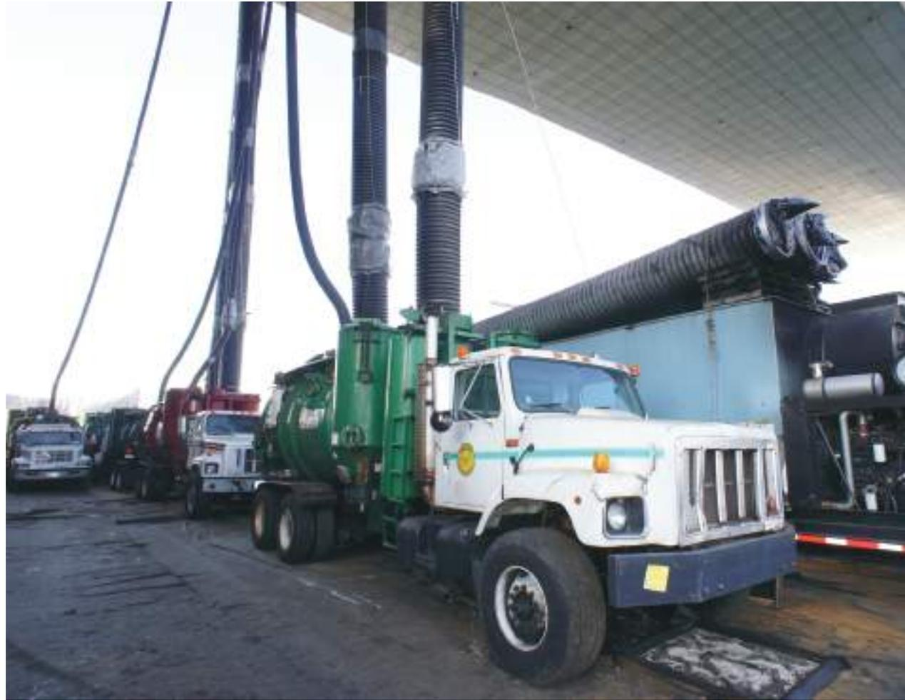
Lead-based paint removal required complete “cradle to grave” handling of hazardous wastes, with equipment situated over 1,200 feet away from the class 1A containment due to weight limitations of the structure and roadway closure limitations.
