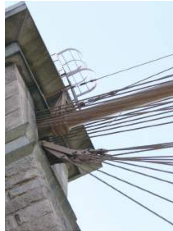
Approximately 4.2 million square feet (390,193m<sup>2</sup>) of steel beams, braces and cables of the bridge, as well as the Manhattan and Brooklyn ramps – essentially the structural “bones” – were specified for a coatings overhaul.
