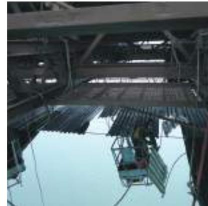
A non-project associated barge and the crane it was transporting struck the under-bridge platform, fortunately causing no injuries, but created a 50-foot-wide (15m) gash which snapped numerous platform support cables, again causing an adverse effect on the CPM; removal of the platform for repair was done as an emergency condition under coordination with the Office of Emergency Management and in conjunction with the SafeSpan design engineer.
